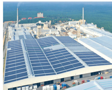
The rooftop distributed PV power at Malacca Industrial Park in Malaysia
