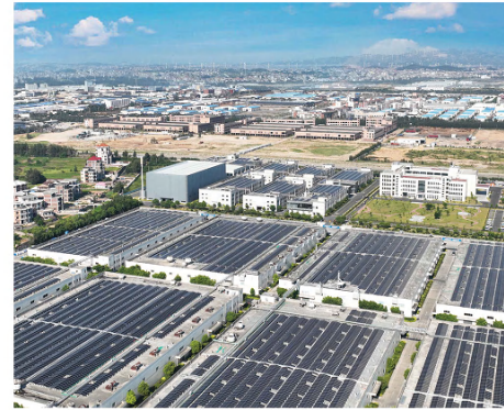
The rooftop distributed PV power plant of Huafeng Group
