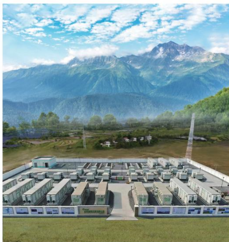
Energy Storage Project in Laohekou,Hubei
